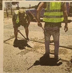
Residents of Koingnaas used more than 50t of concrete to fix the potholes in their town.
